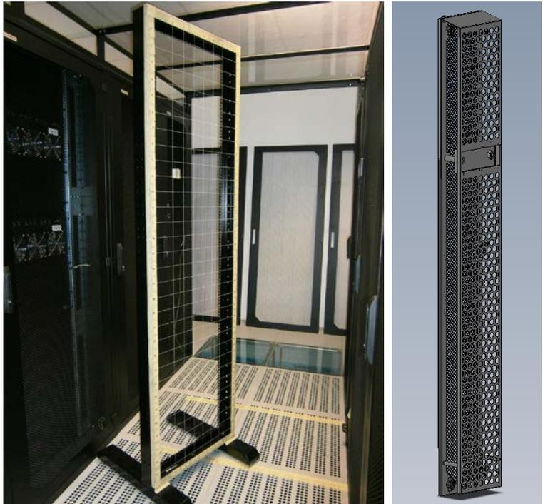
The measurement at the air intake of the cooling unit has shown that the change of air-flow will not be significant. The more narrow rim on the front door frame is not so big change to see dramatically increased air-flow.
